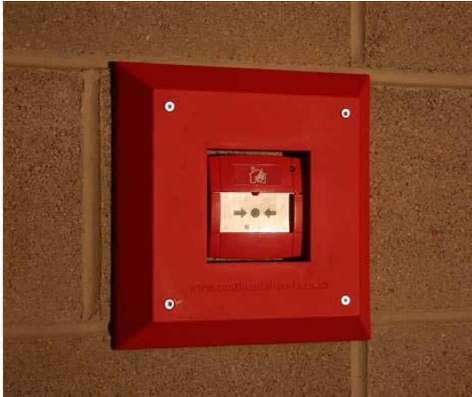
**Figure 3: Protective shielding for Manual Call Points**
