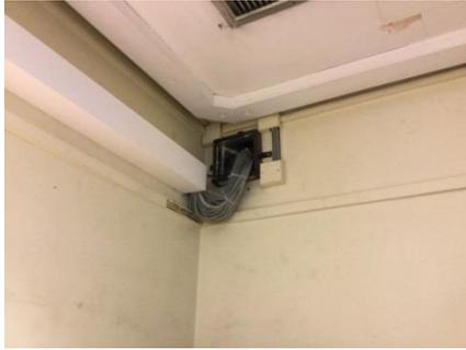
(Img 4): Inadequate fire-stopping of service penetrations is a prevalent defect observed during inspections of passive fire protection.
