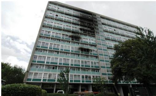
(Img 1): The west face of Lakanal House showing the extent of fire spread, which started on the 9th floor, spread up to the 10th and 11th and dropped down to the 5th and 7th floors.
