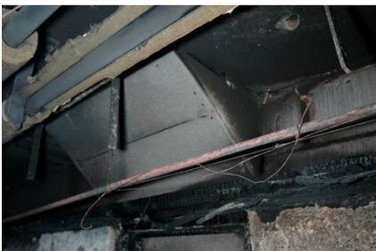
(Img 2): Fire damaged "boxing in" along the 11th floor corridor at Lakanal House.
