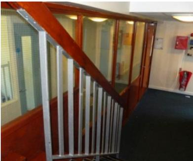
(Img 3): Old style Georgian wire glass partition being used to protect escape staircase. Favoured in the past for its physical integrity, this type of glass provides little barrier to flame radiation and can allow fire to quickly penetrate.
