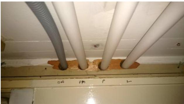
(Img 2): Retrofitted services pushed through a fire rated door frame, rendering the existing fire rating ineffective.
