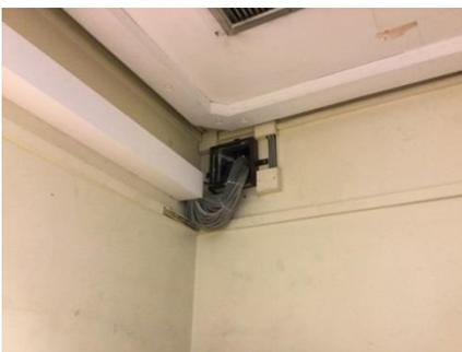
(Img 4): Inadequate fire-stopping of service penetrations is a prevalent defect observed during inspections of passive fire protection.
