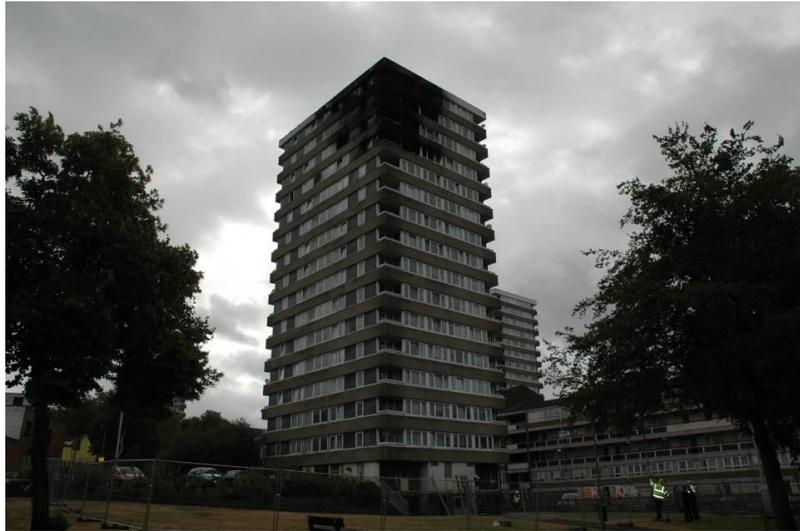
**Figure 1 – Block of flats showing extent of fire damage caused by holes in compartmentation on balconies**
